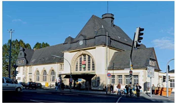
Passenger building of Friedberg station in Hessen after energy-efficient renovation
